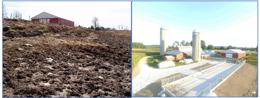
From left to right, before and after photos of heavy use area protection implementation.
